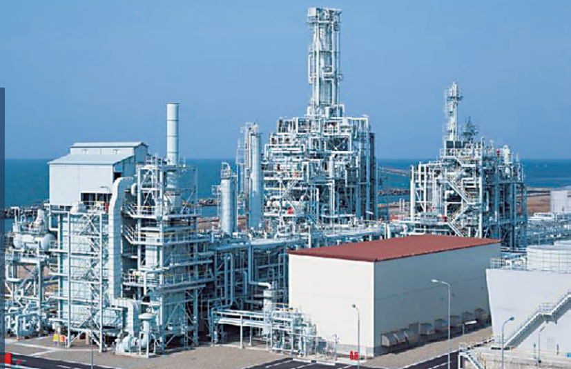
GTL demonstration plant (photo courtesy of Nippon GTL Technology Research Association)
